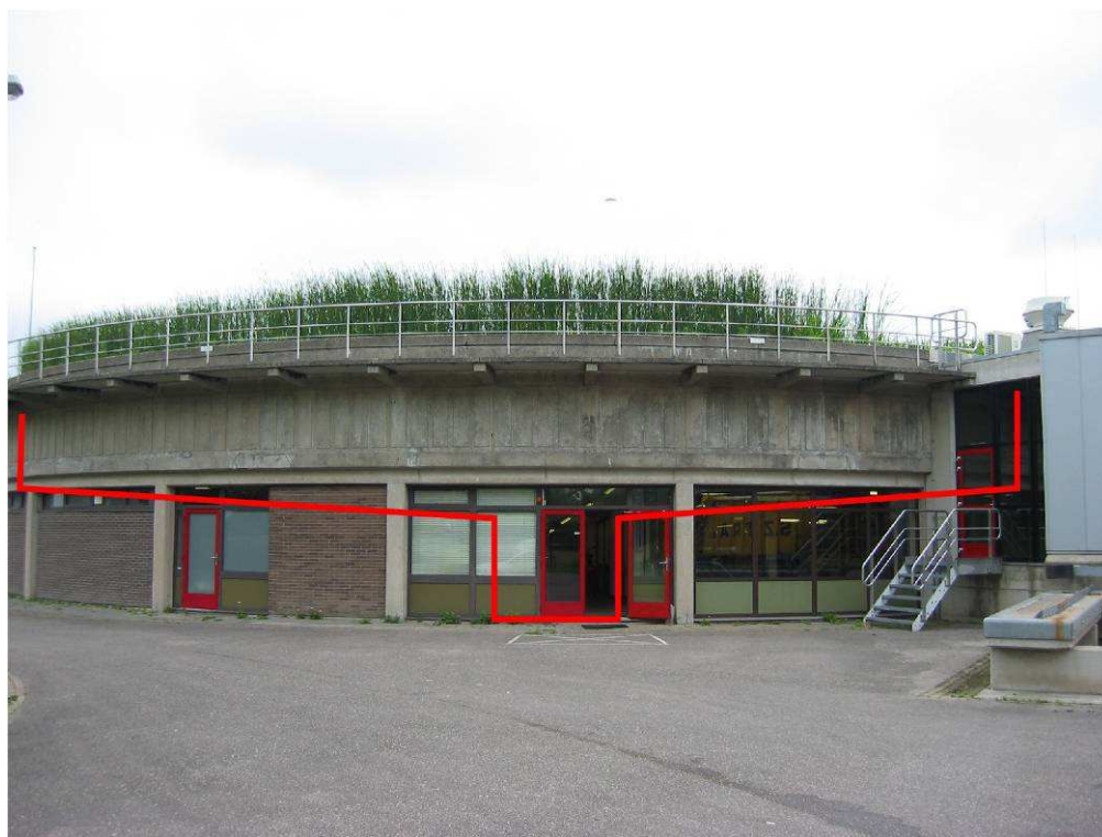
image 2.1 Side view of one of the basins.
