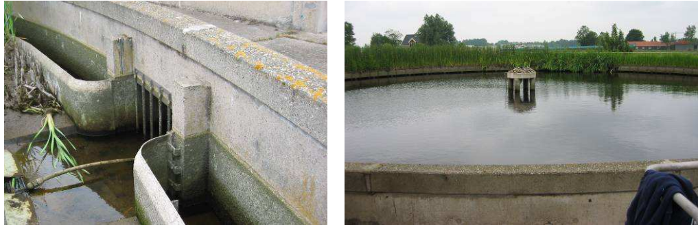
image 2.2 View of the tunnel and an image of one of the basins.
