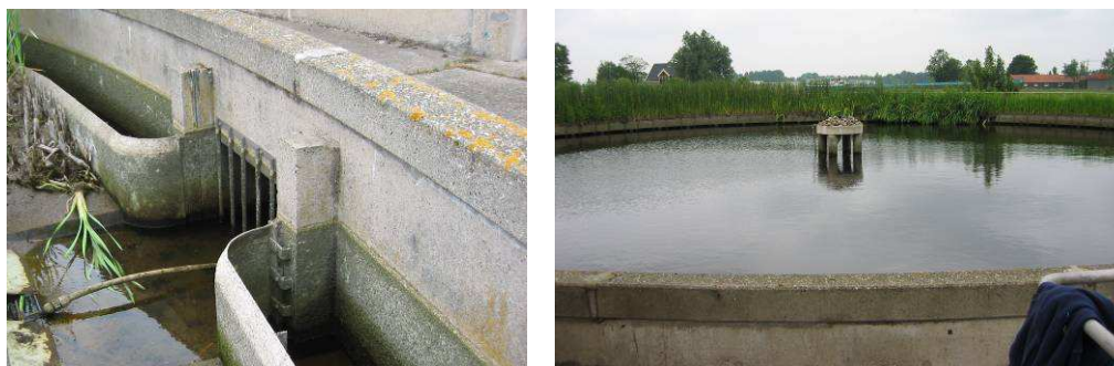
image 2.2 View of the tunnel and an image of one of the basins.
